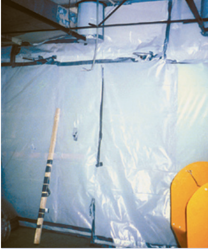
Photo 8: Full containment on large job
